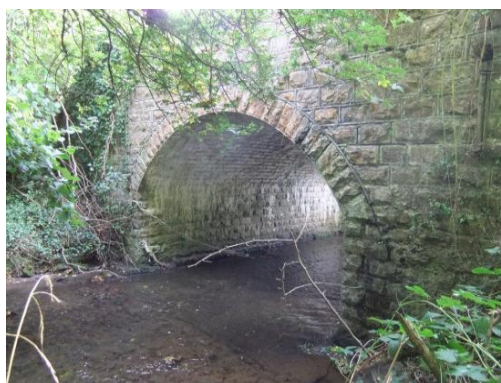
Figure 15.6 Five Mile Lane crossing the River Waycock
