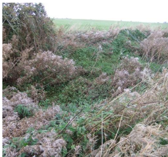
Figure 15.13 Ford Brook downstream of Five Mile Lane
