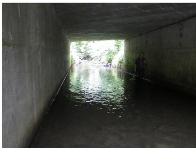
Photograph 5. Deep dark water beneath the road bridge.
