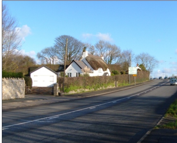
Plate 1: Sheepcourt Cottage. View from the west
