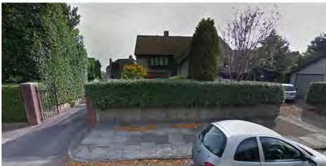
2 Storey House - cream/ grey brick with timber bay and pantile concrete gable roof- circa 35' pitch, dwarf wall to front boundary with hedge
