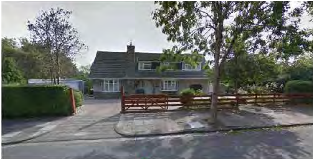
Single storey Dormer Bungalow in render with stone detailing, white windows bay features, grey concrete tiled roof (38 degree pitch), Timber picket Fence
