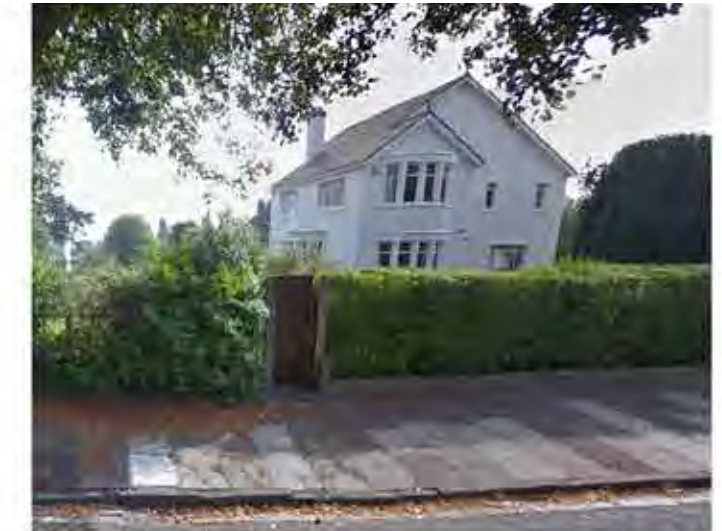
Large white rendered house – with bay window to front, gabled slate roof 30' pitch volume 1705m3 note this house is 2.4m higher than building B. Hedge boundary treatment
