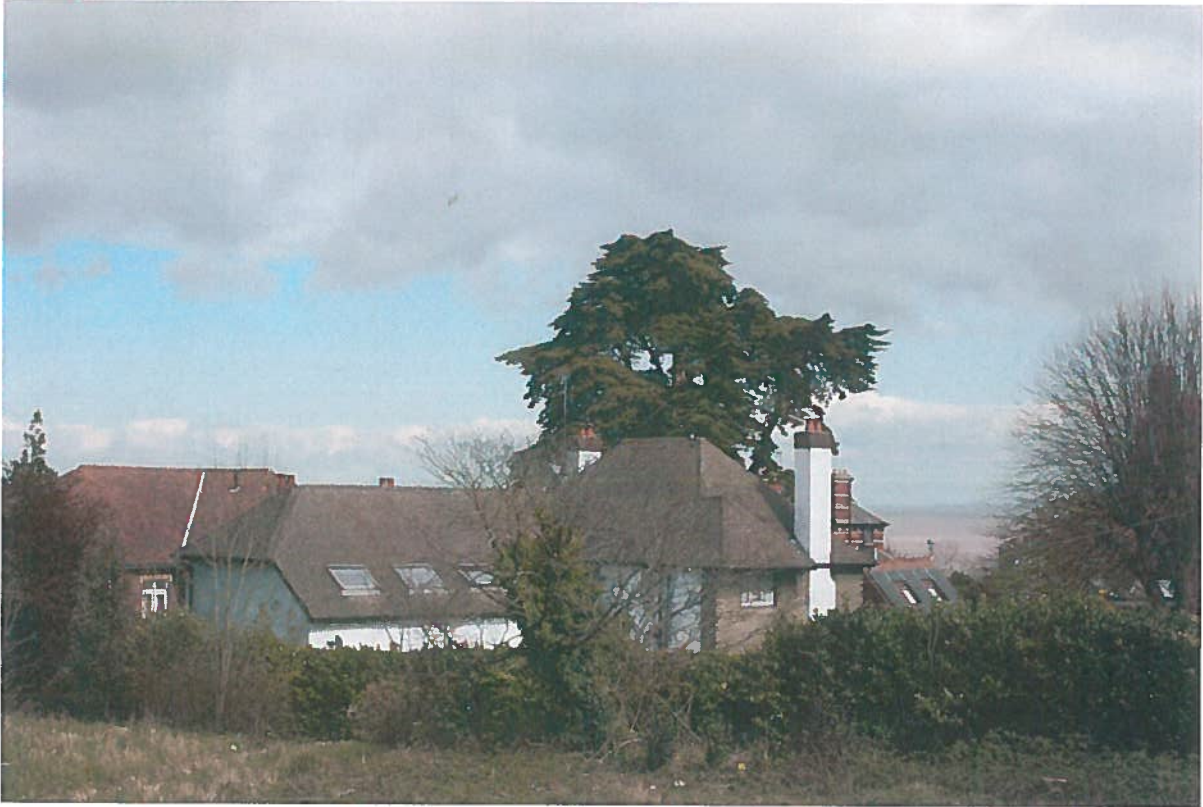
Image EDP 7: Typical view east from the site and illustrating the diversity of building and roof forms in the adjoining parts of the Penarth Conservation Area.
