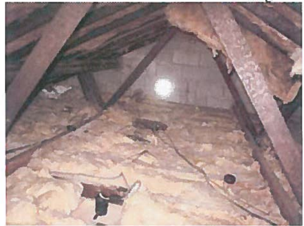
Attic void above extension
