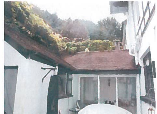
View of outbuilding
