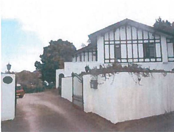
View of western elevation Northcliffe Lodge
