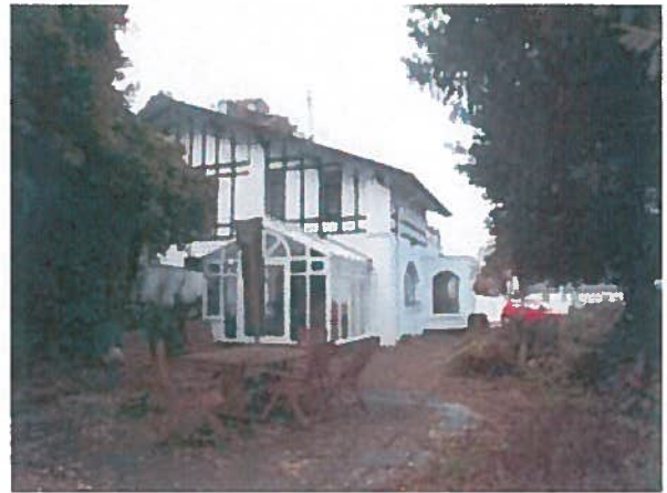
View of eastern elevation Northcliffe Lodge
