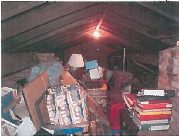
Attic void in main house
