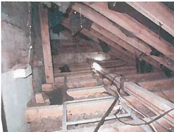
Attic void above outbuilding
