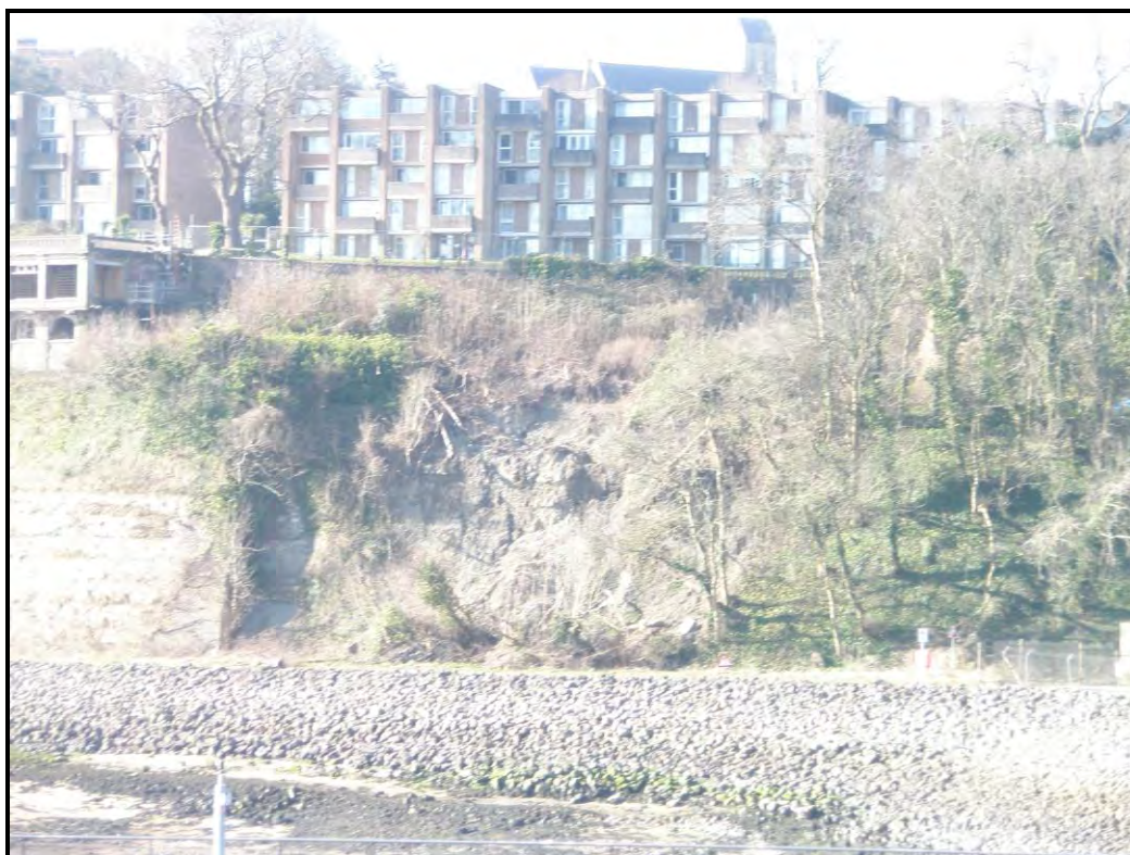
Plate 2.2. 2013 Landslide adjacent to study site.
