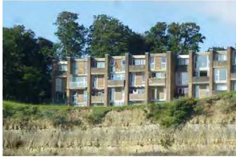
Below: North elevation of brick built Northcliff Flats, (circa 1970's)
