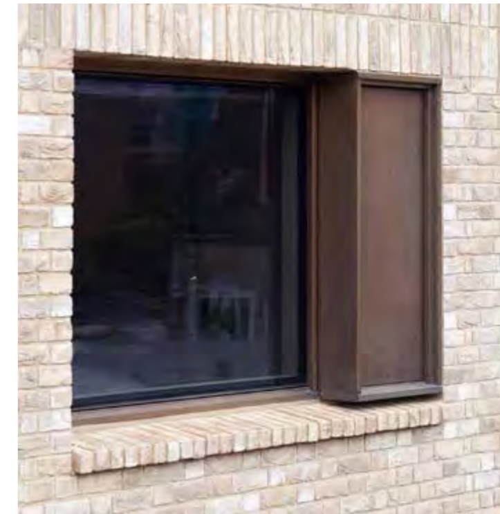
above: operable shutters/insulated panels are proposed to animate the elevations and provide individuality between apartment types
