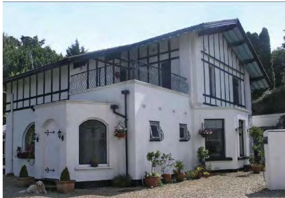
Below: The existing Northcliff Lodge (circa 1940's) including rear extension addition, entrance gateway and linking elements
