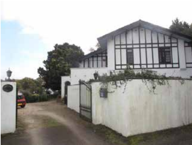
View of western elevation Northcliffe Lodge
