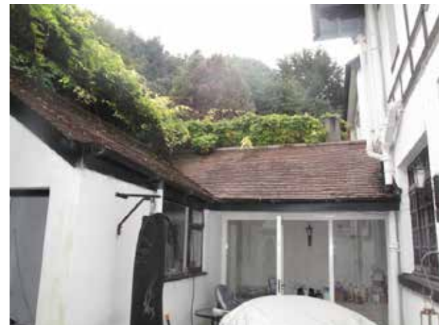
View of outbuilding
