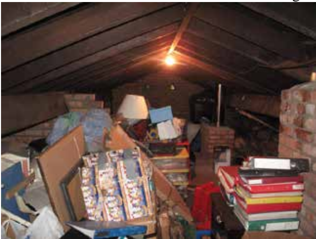
Attic void in main house
