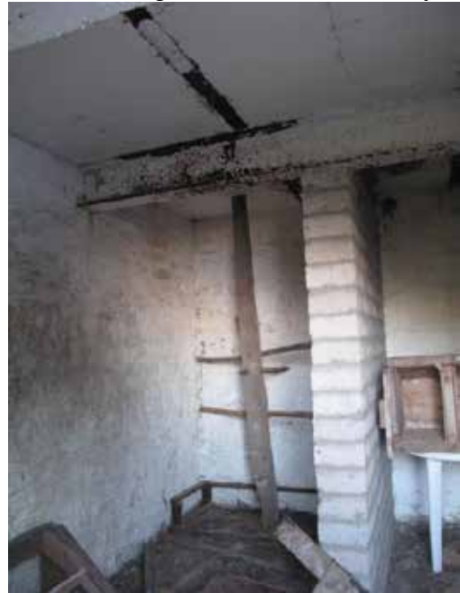
Example of shed interior
