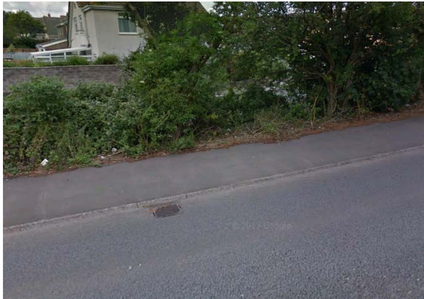
Figure 2-2 View of the South Road adjacent to the Site depicting gully trap
