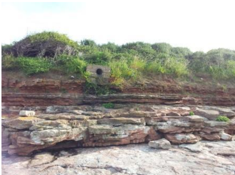
Figure 11: Outfall headwall from unidentified surface water outfall
