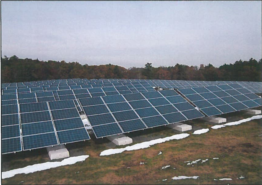
Figure 1: Photograph of Typical Mounting Details (N.B. indicative of mounting details only)
