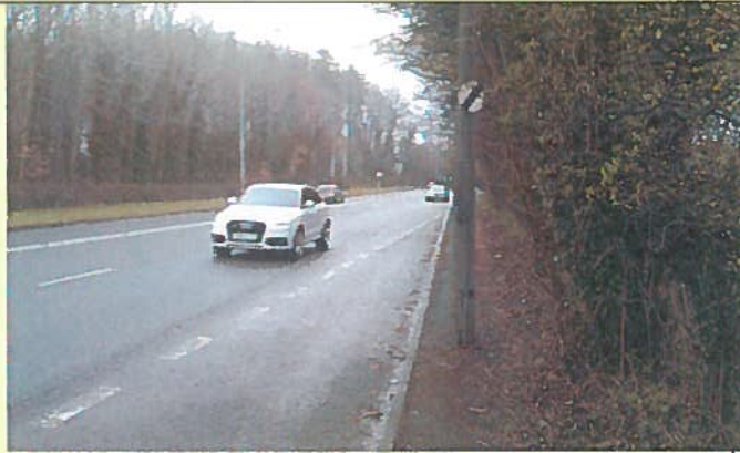
Tumble Hill, A48 - inadequate footpath obstructed (2015)
