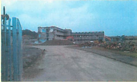
Media Centre demolition = Less employment
