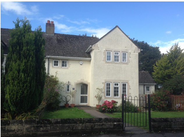
Example of off-white rough render and architectural details such as corbels and quoins on estate housing in St Nicholas
