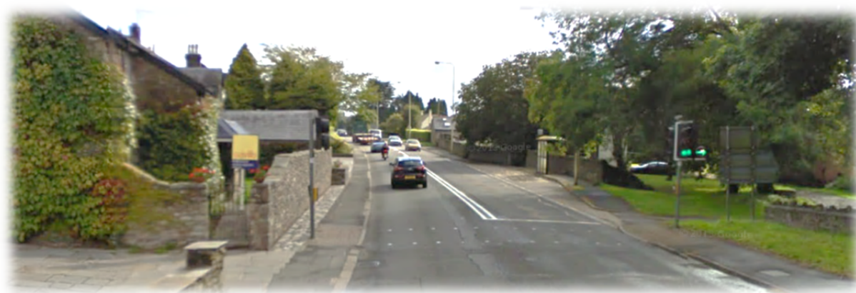
Photograph 1 – A48 and pedestrian crossing facility
