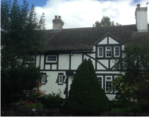
White rough cast render and black detailing around windows and black timber work are seen occasionally within the village.
