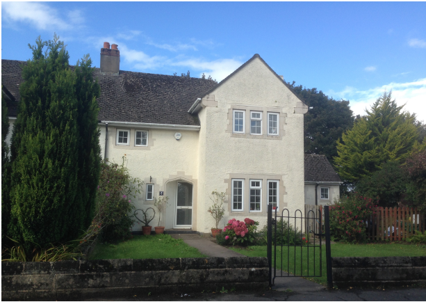
Example of off-white rough render and architectural details such as corbels and quoins on estate housing in St Nicholas
