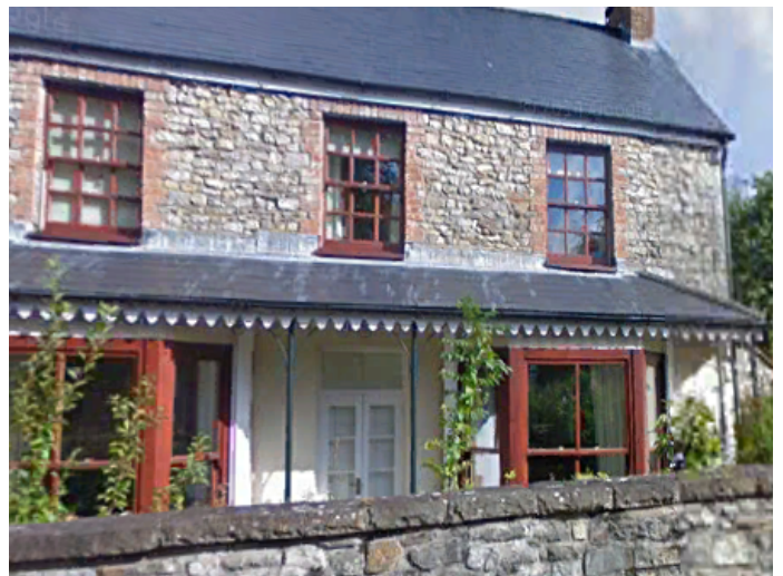
Example of brick accents around windows in St. Nicholas
