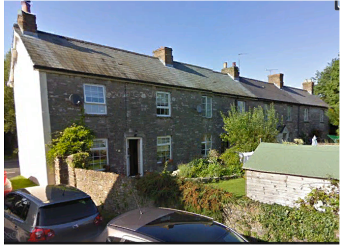
A row of terraced cottages in stone, with the use of render on other building elevations.
