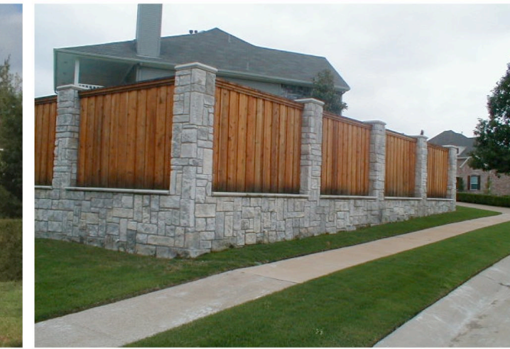
Stone wall with fence panel & piers
