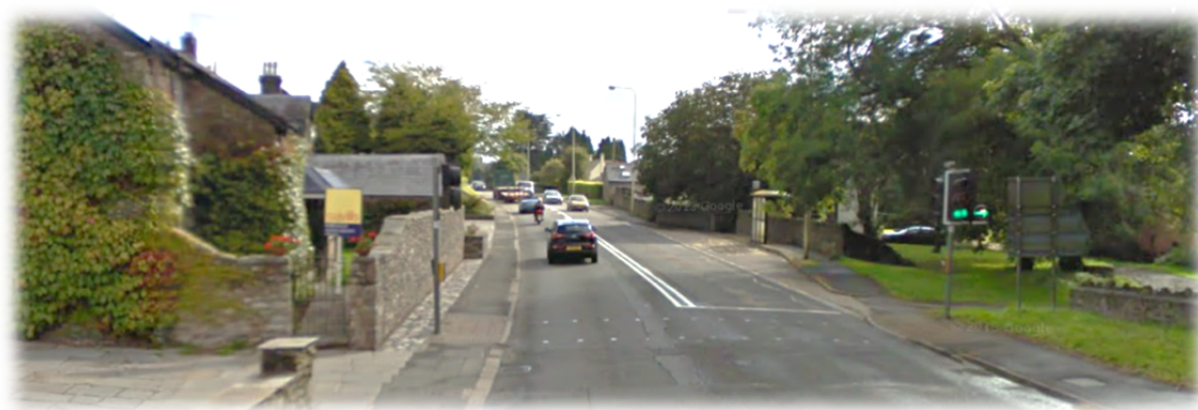
Photograph 1 – A48 and pedestrian crossing facility
