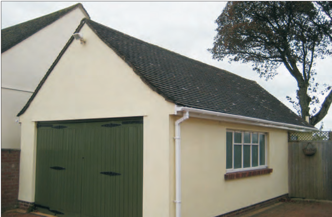
PHOTOGRAPH 5: View of Building B2
