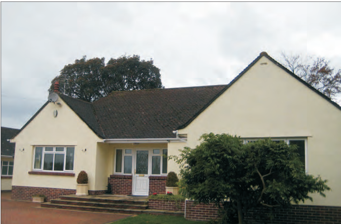
PHOTOGRAPH 4: View of Building B1
