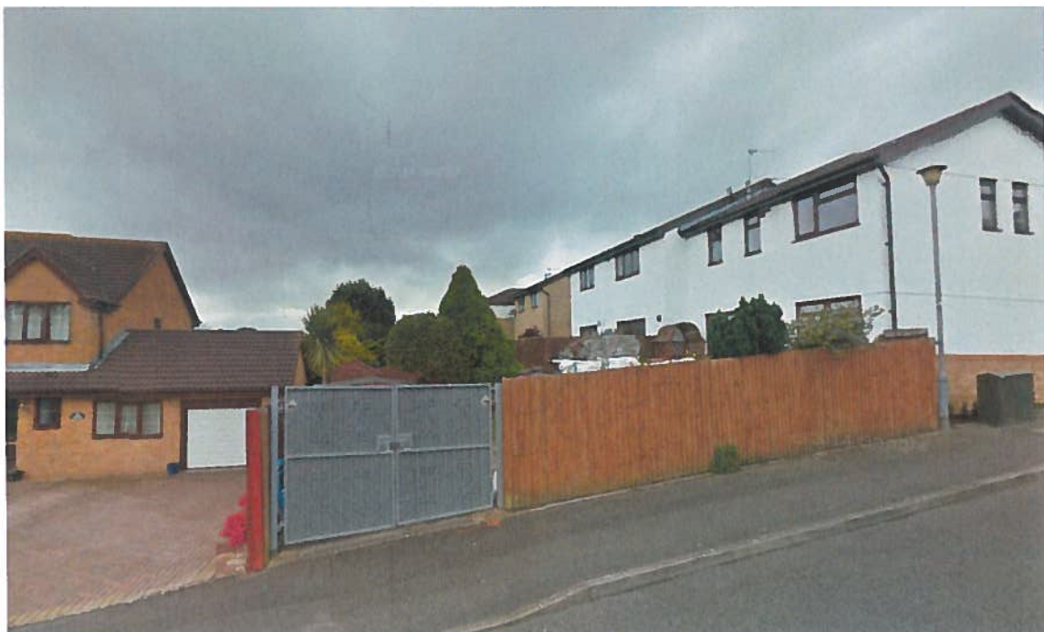
Existing Side view from Priory Garden
