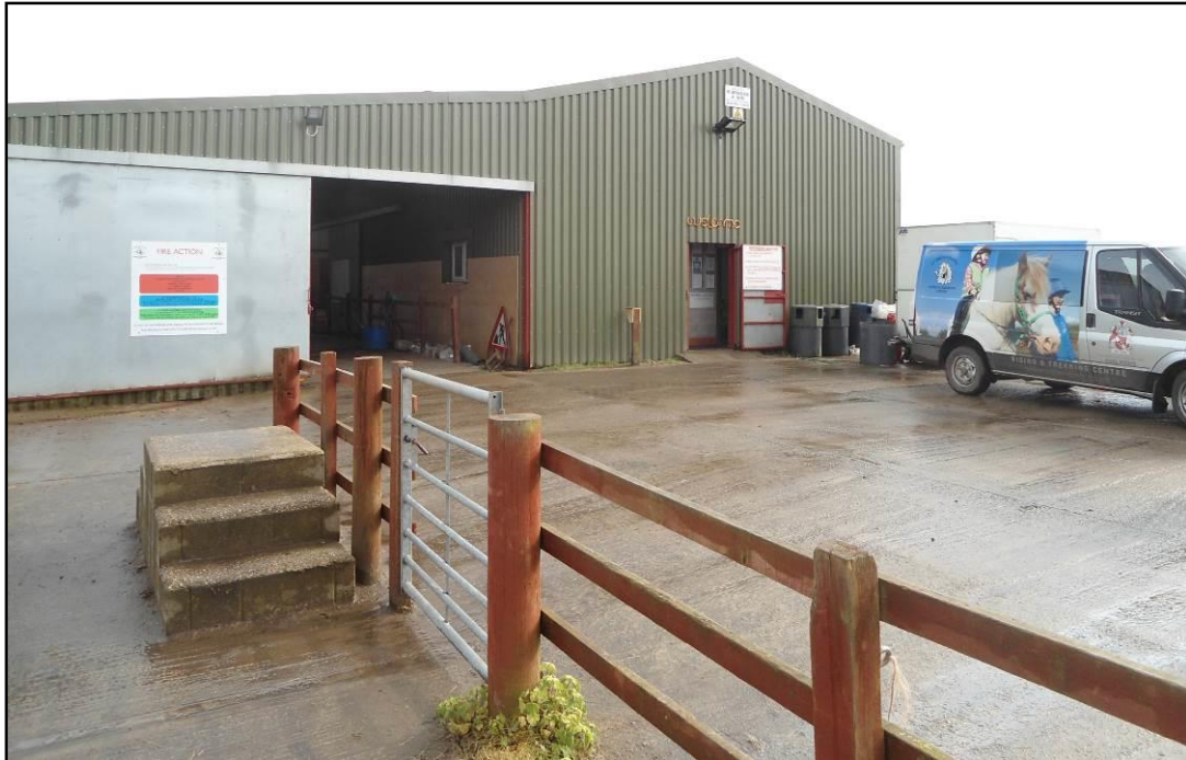
Figure 3. The proposed building would be a similar external appearance to the existing building.
