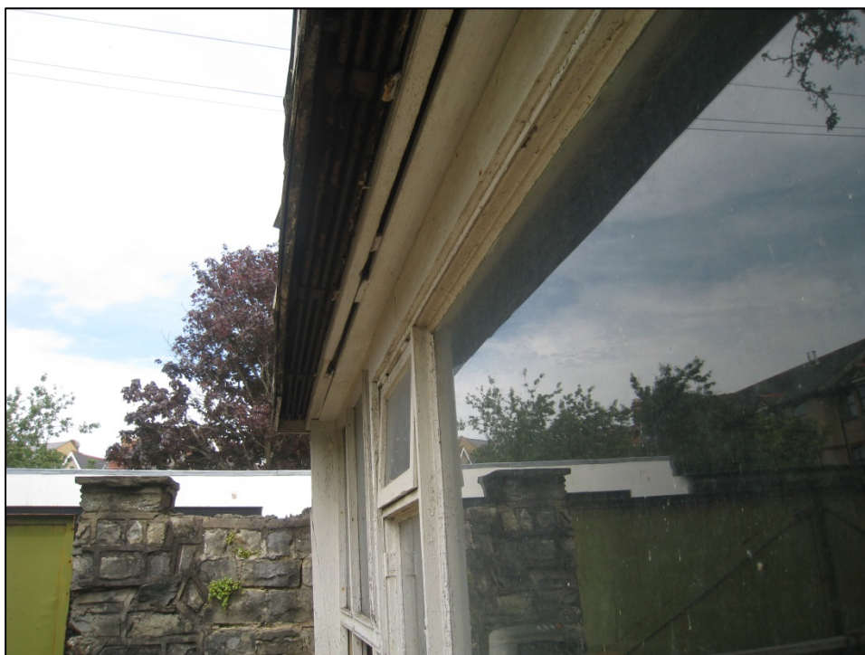
Plate 2 Timber cover for metal bracket of former roller door or awning
