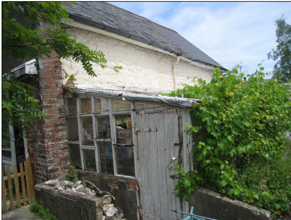
Plate 2 Timber cover for metal bracket of former roller door or awning
