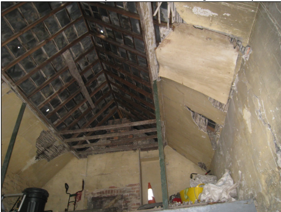
Plate 4 Interior of Coach House – Exposed roof slates and damage to lathe & plaster ceiling
