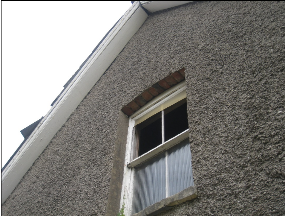
Plate 3 Window in western gable and gap in fascia at apex of gable end
