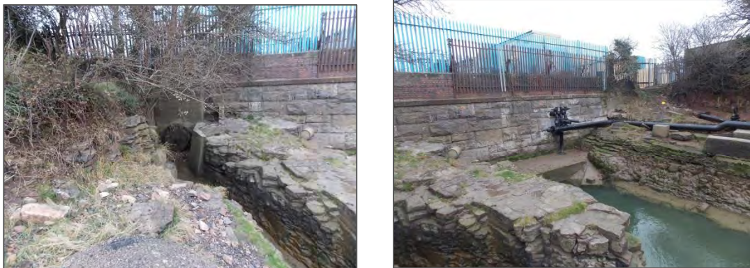
Figure 3: Cadoxton Sea Outfall (sluice gate) and the Cadoxton River embankment
