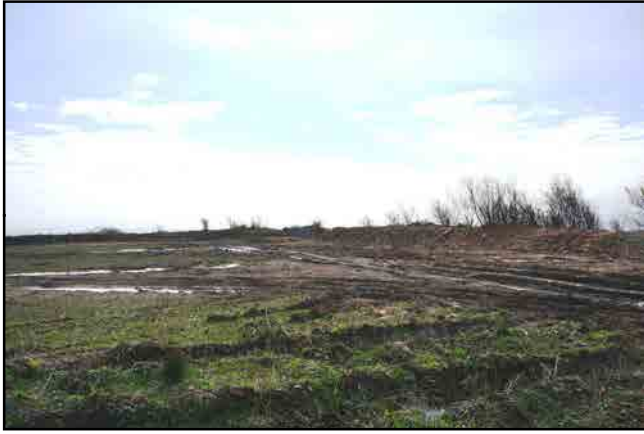
Photograph 7: Disturbed ground of ESP3 showing machine tracks with pooled water.
