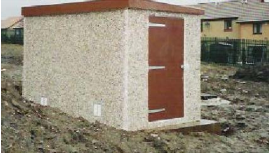
Image 4. Image of the potential switch gear container
