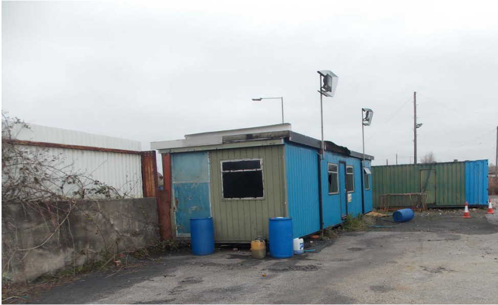
Image 5. Single story portable building to be demolished as part of the proposed works
