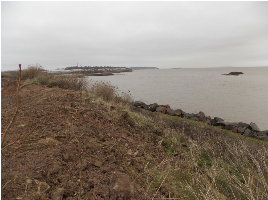
Image 1. An example of bunding on the perimeter of the redline boundary
