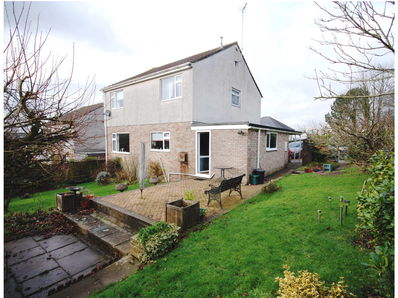
South / Rear of property
