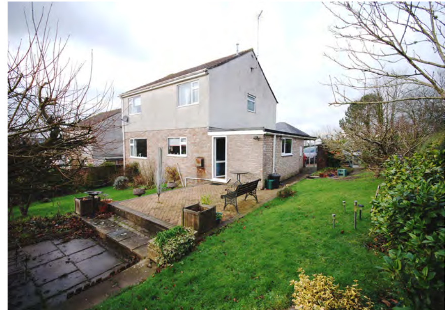
Rear Elevation. The Garage is to be part demolished for the extension
