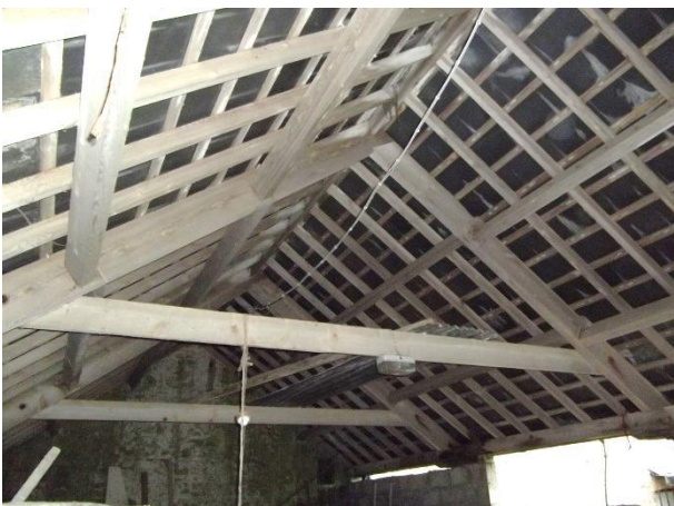
Figure 6 – internal view of building D;
