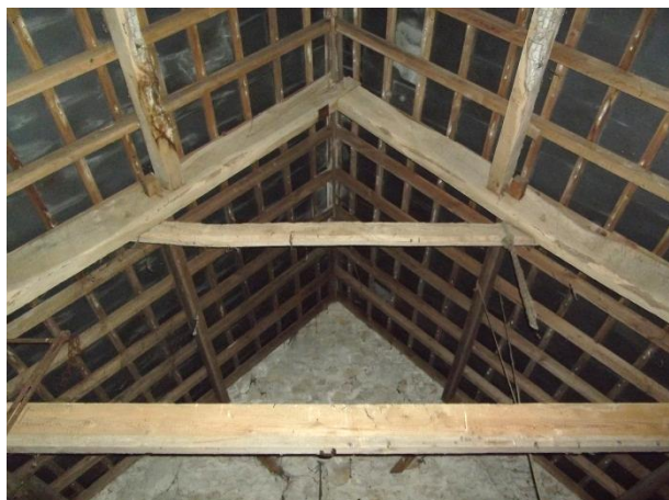
Figure 8 – internal view of upper floor within building E;
