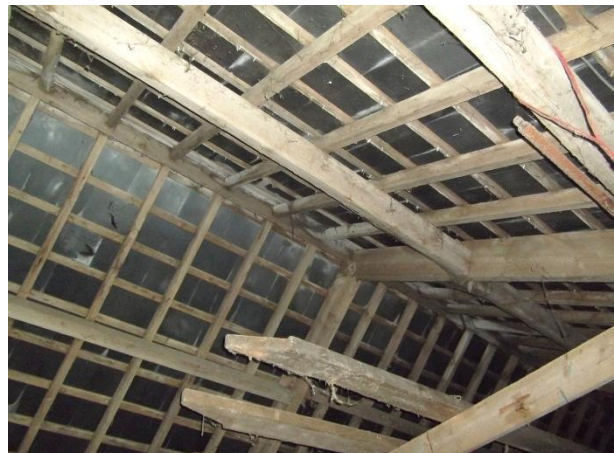
Figure 5 – internal view of building C;
