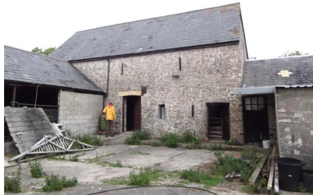
Figure 3 – building E as viewed from the west;
