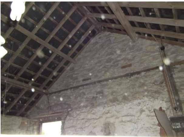
Figure 4 – internal view of building B;
