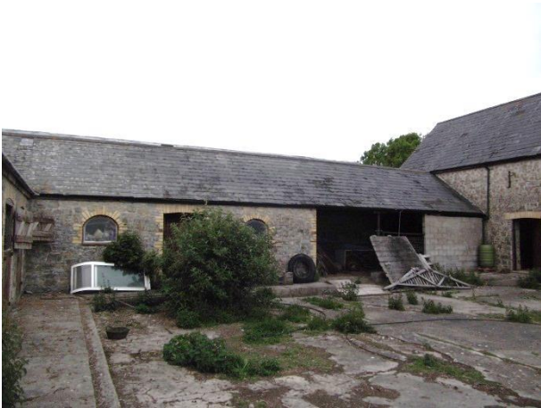
Figure 2 – buildings C and D as viewed from the south;
