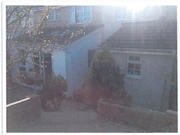
Image 4 Existing North Elevation showing rear extension
