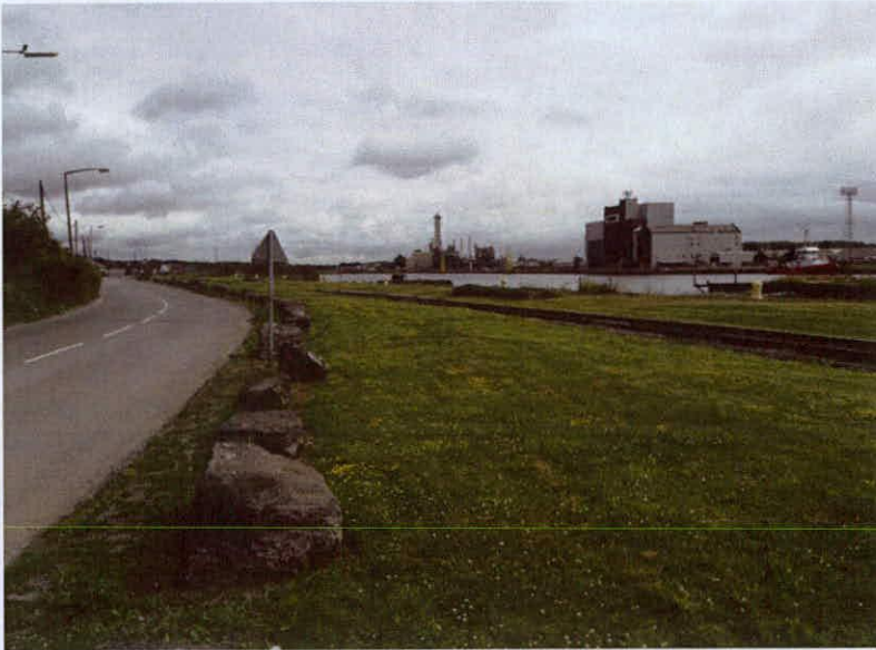
8. South boundary looking east
