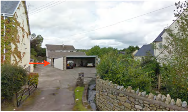
Existing access (indicated by the red arrow) is via Sydney House Farm yard and tucked behind a carport.
