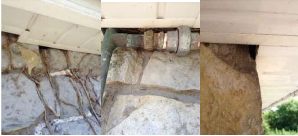
Fig. 8-10 Potential bat access points into soffits of garage/extension
