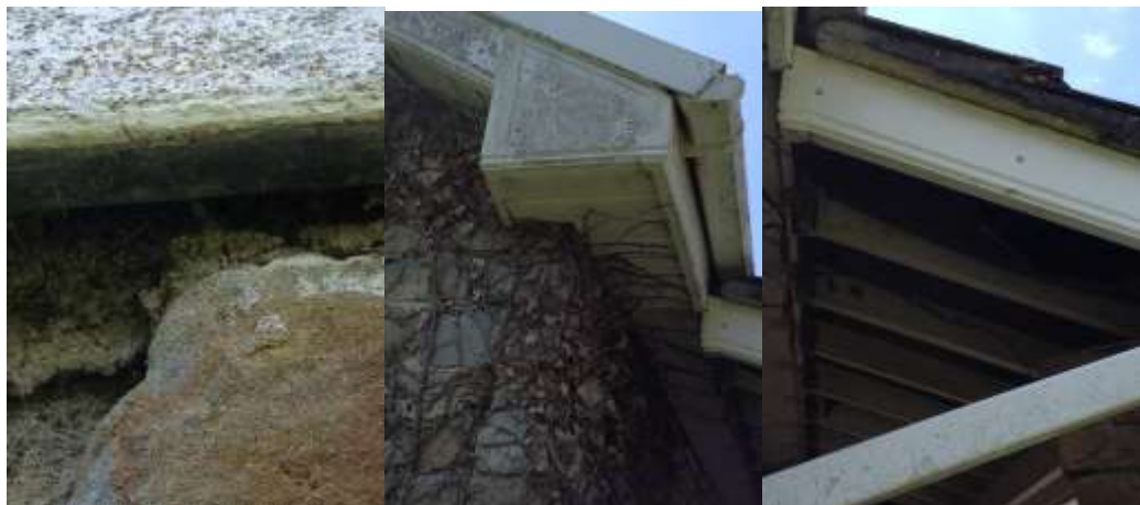
Fig. 11-13 Potential access points on the garage extension/veranda
