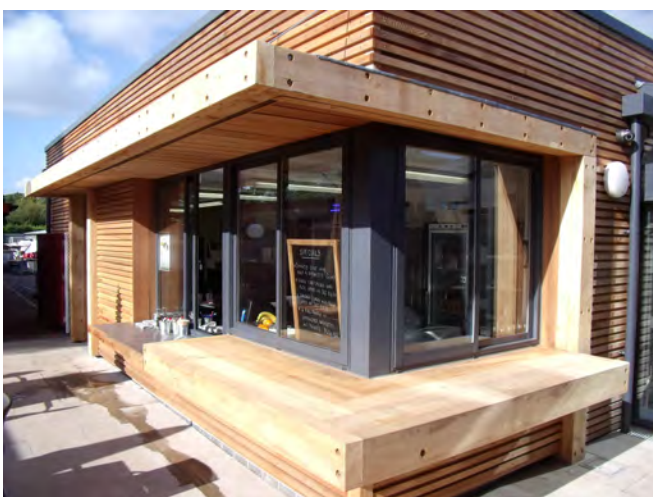
Timber framing is proposed to windows as shown here at the Bute Park Nursery building, Cardiff
