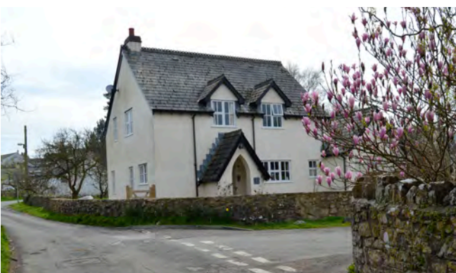
The Pump House is located opposite Black Barn House
