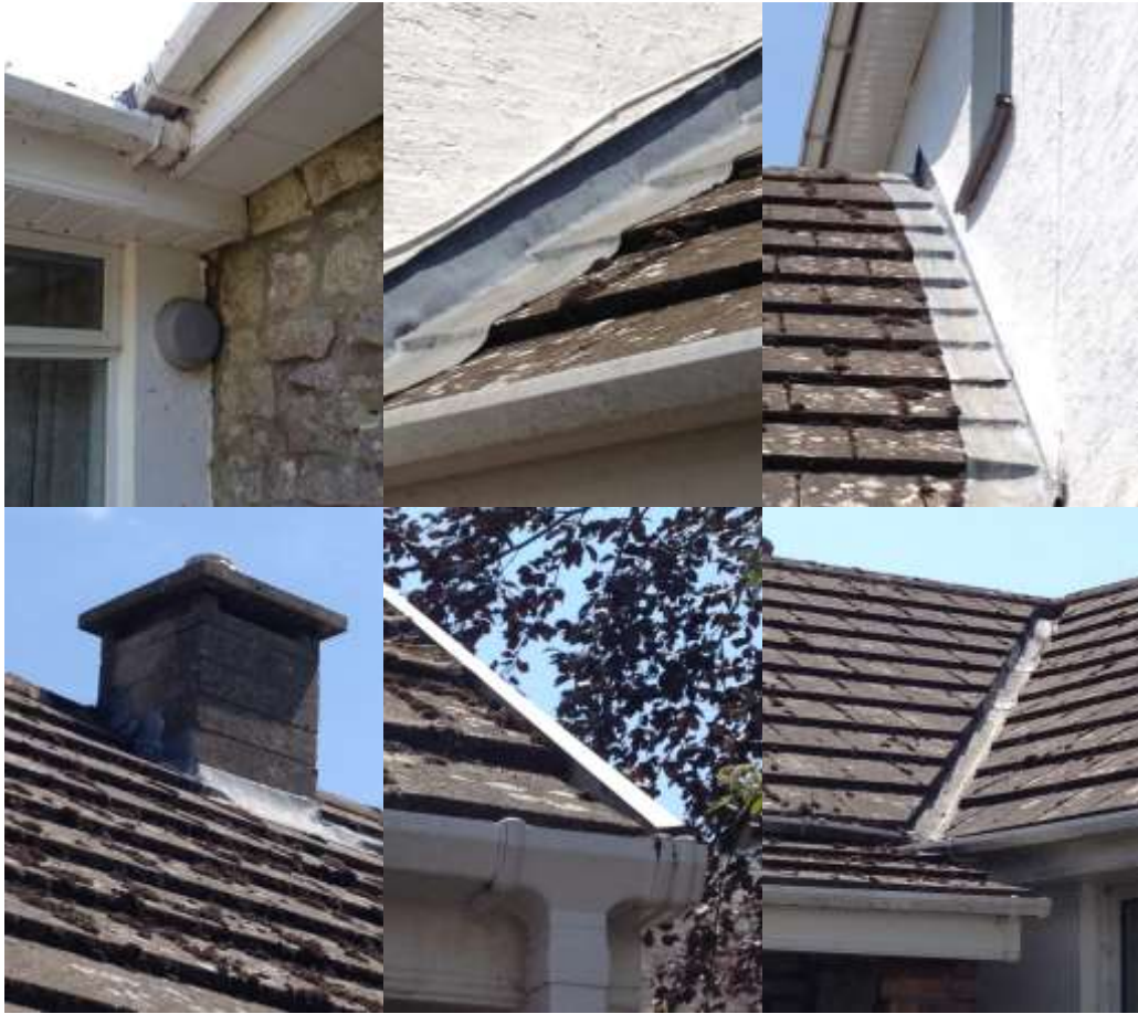
Fig. 22-27 Ridge and roof tiles in good order
