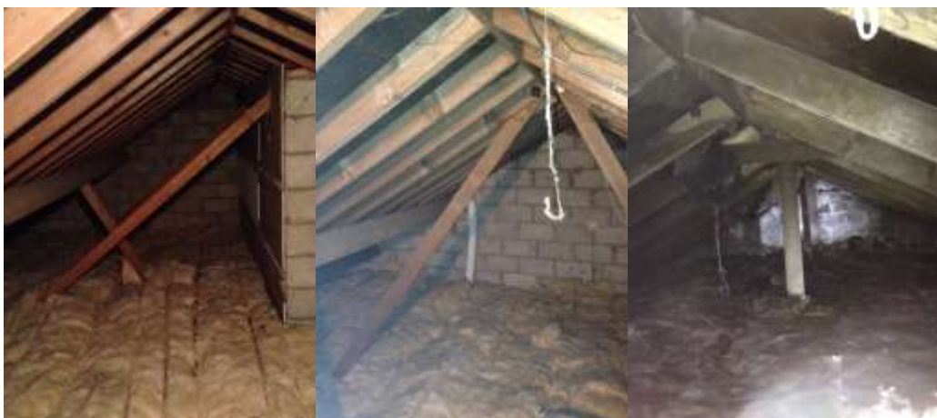
Fig. 28-30 Roof beams and sarking in good order
