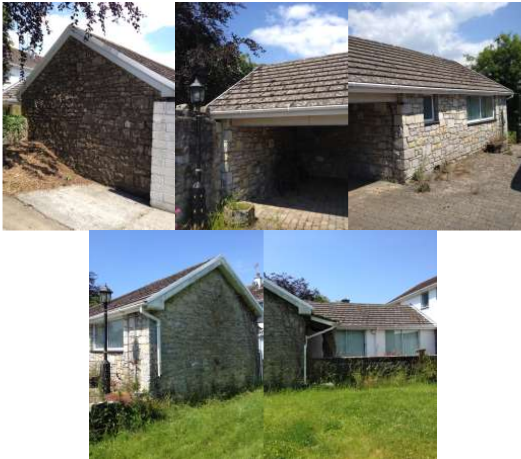
Fig. 3-7 Garage/parking bay and single-storey extension
