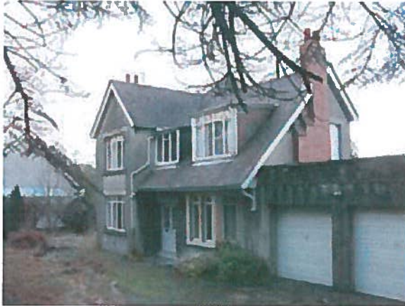
Front (west) elevation of the house
