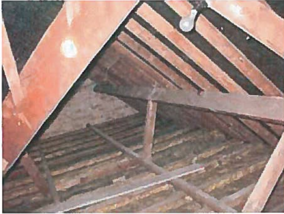
Interior of roof void
