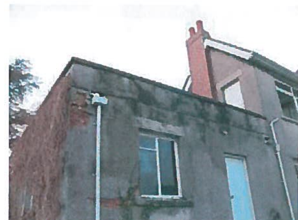
Adjoining garage present on south elevation
