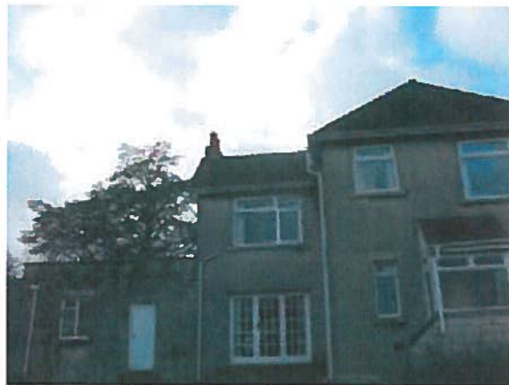
Rear (east) elevation of the house
