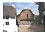
12 The Neck, Ormskirk Use of sensitive materials to enhance the local character
