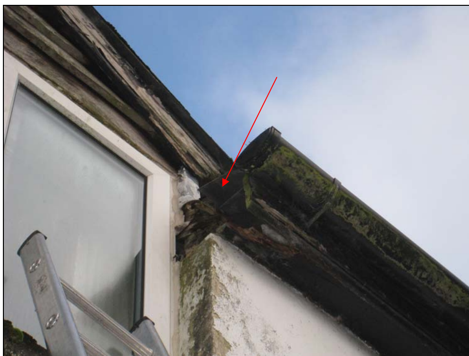
Plate 1. Gaps in southern elevation soffit with bird nesting material found within space
