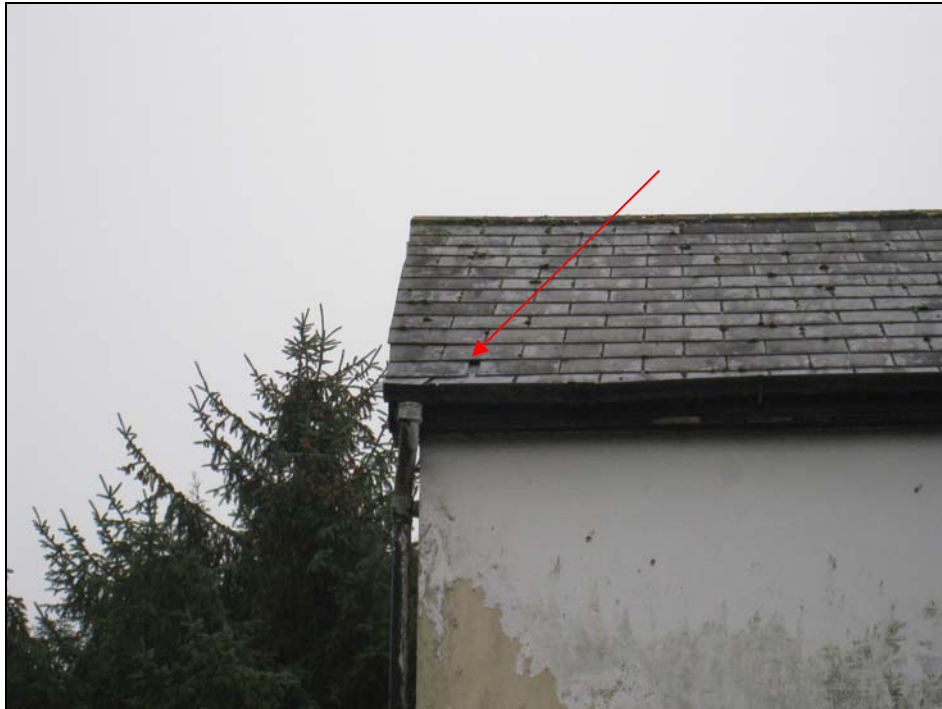
Plate 4. Gap in roof tile on northern elevation
