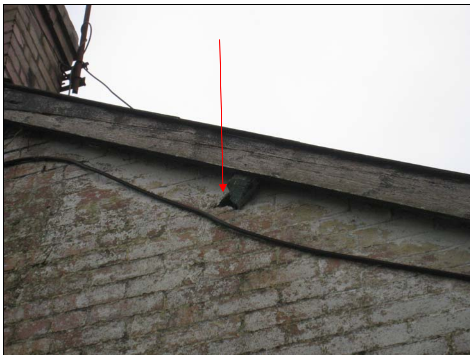
Plate 3. Missing brickwork/render where the structural timbers protrude from the gable end
