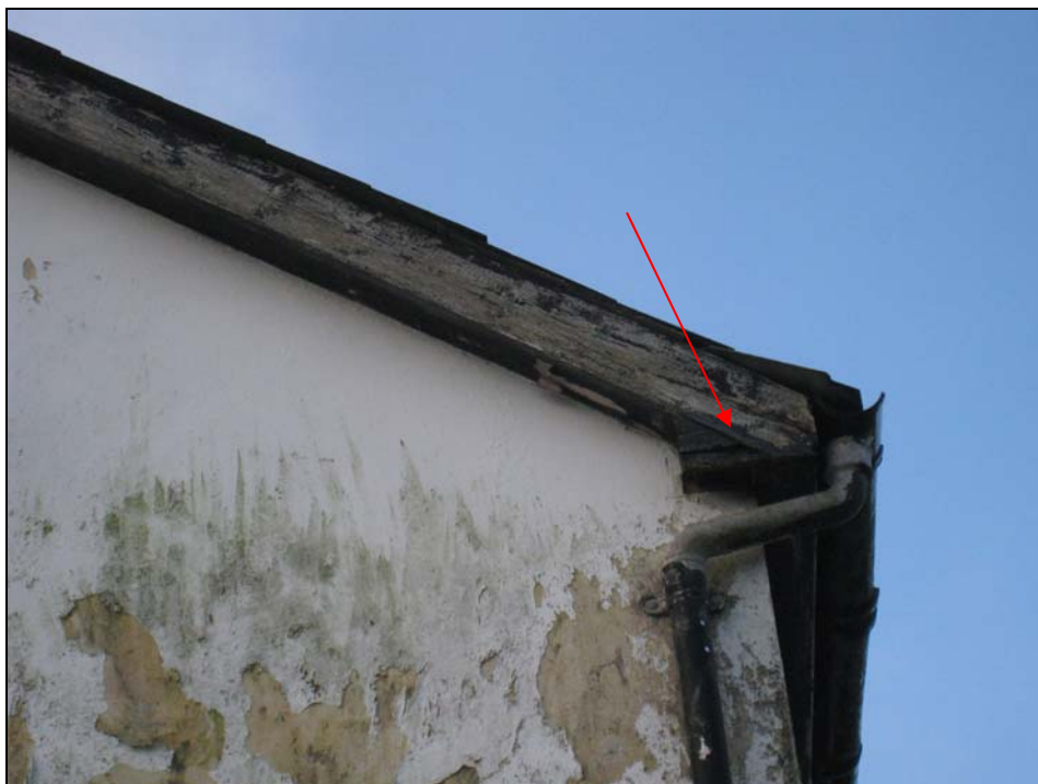
Plate 5. Gap in the fascia on the north east corner of building
