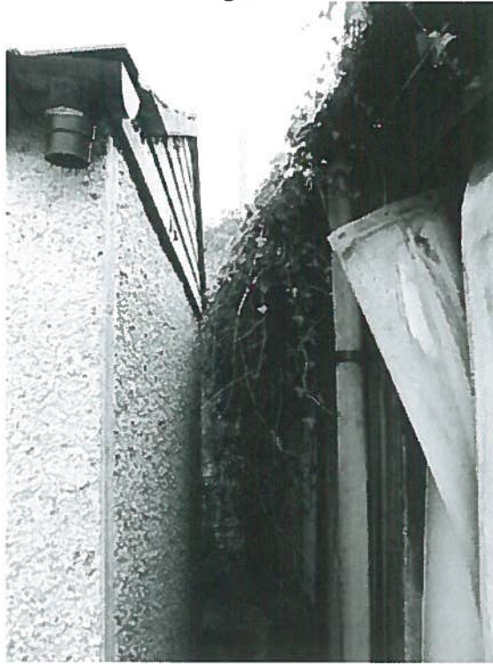
East gable end
