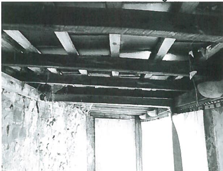
Roof void of out building
