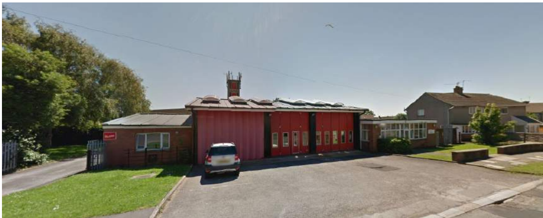
Existing Building Front Elevation
