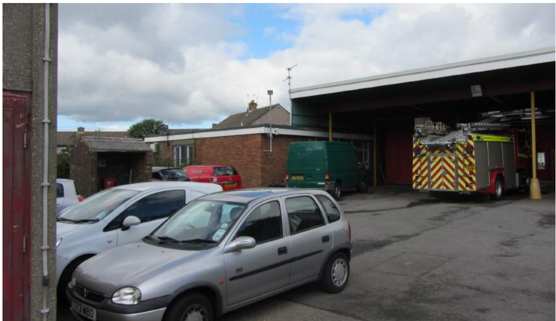
Rear of Fire Station
