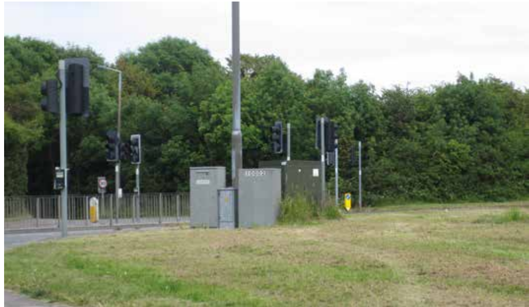
TRAFFIC LIGHTS BETWEEN EGLWYS ROAD AND B4265
