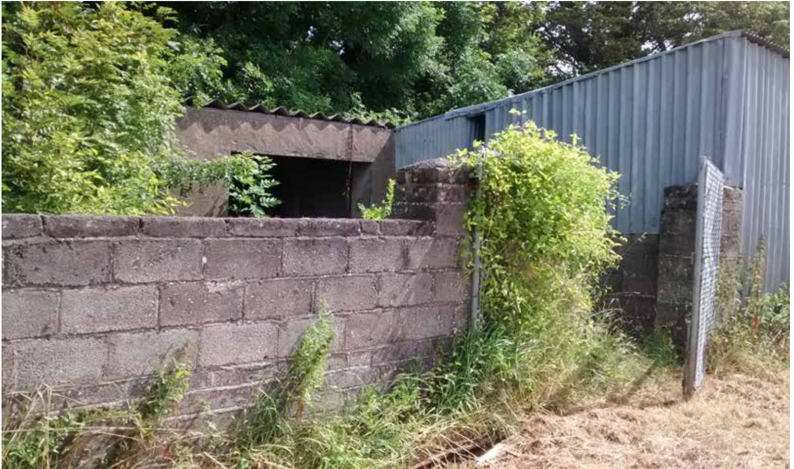
BUILDING ADJACNT TO THE NORTH-EAST BOUNDARY OF THE SITE
