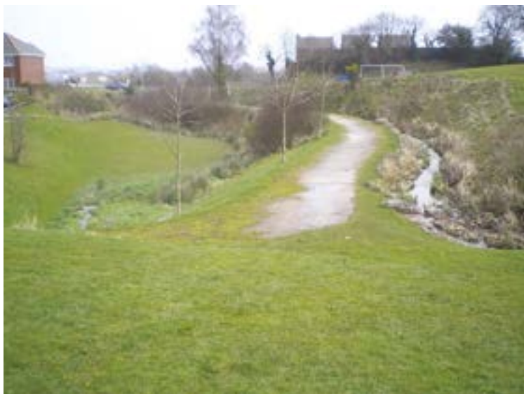
39 | Sustainable drainage systems at Pontyclun
