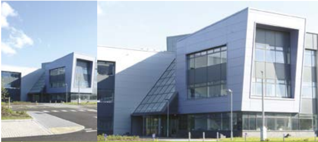
48 | Neath Port Talbot County Borough Council Offices, Baglan Energy Park
