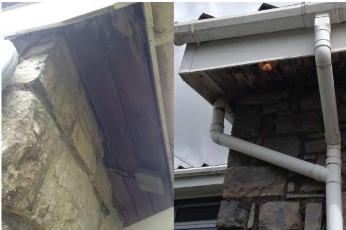
Fig. 18&19 bat access to soffit box
