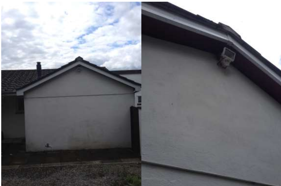
Fig. 6 &7 Two views of rear gable & security light for drive
