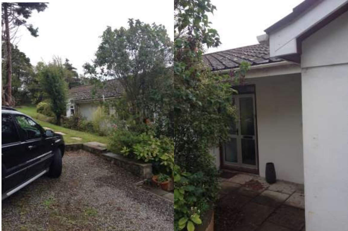
Fig. 2 & 3 Views of the rear of the property including main entrance
