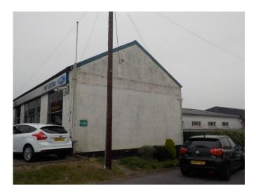
3.8 The proposal therefore is to overcome this issue and enhance the appearance of the building to reflect its status as a car sales garage and install silver colour coated steel profile sheeting to the majority of the external elevations.
