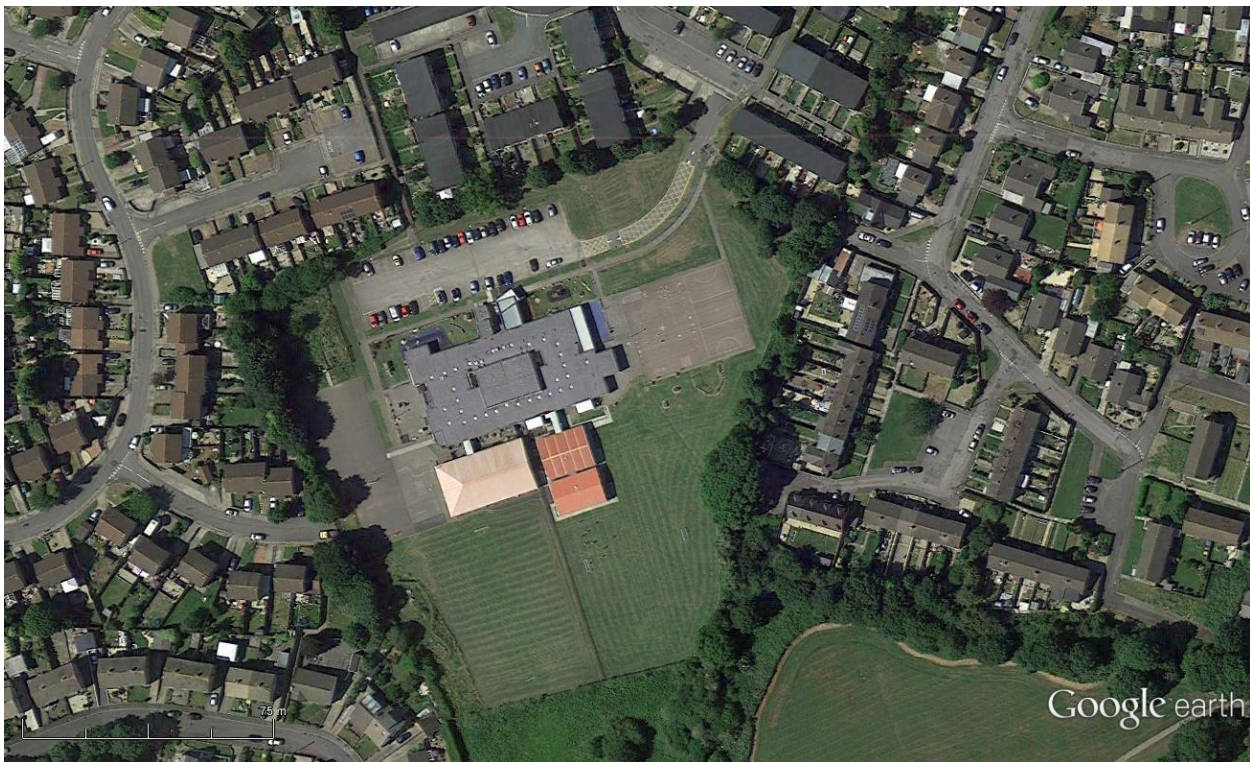
Figure 1 - Aerial image of the Site . NB Image used under licence (© Google 2014).
