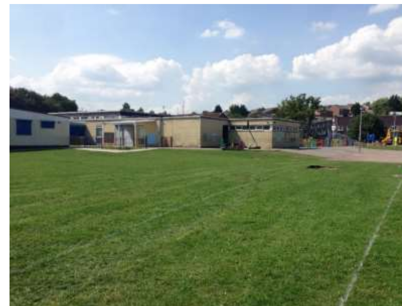
Figure 06 - Existing school building
