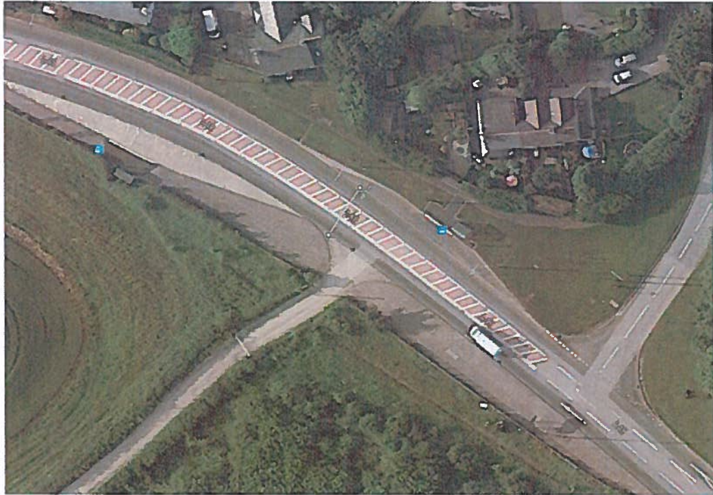
A48 / Llangan Road Junction
