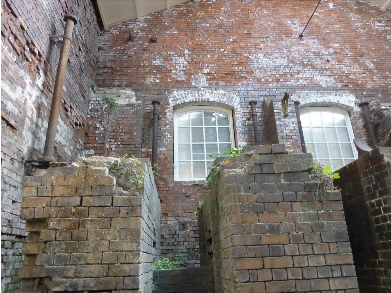
PH24 – east wall of South Range
