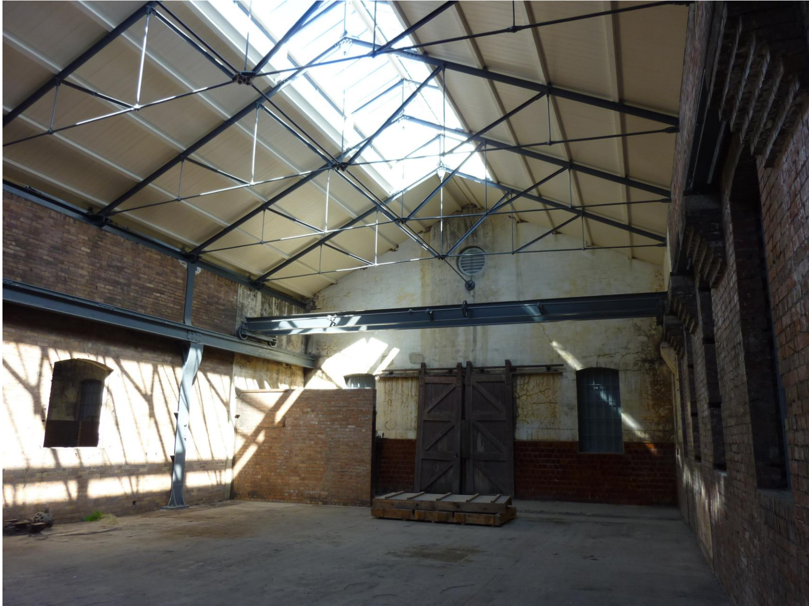
PH8 – north wall of the North Range
