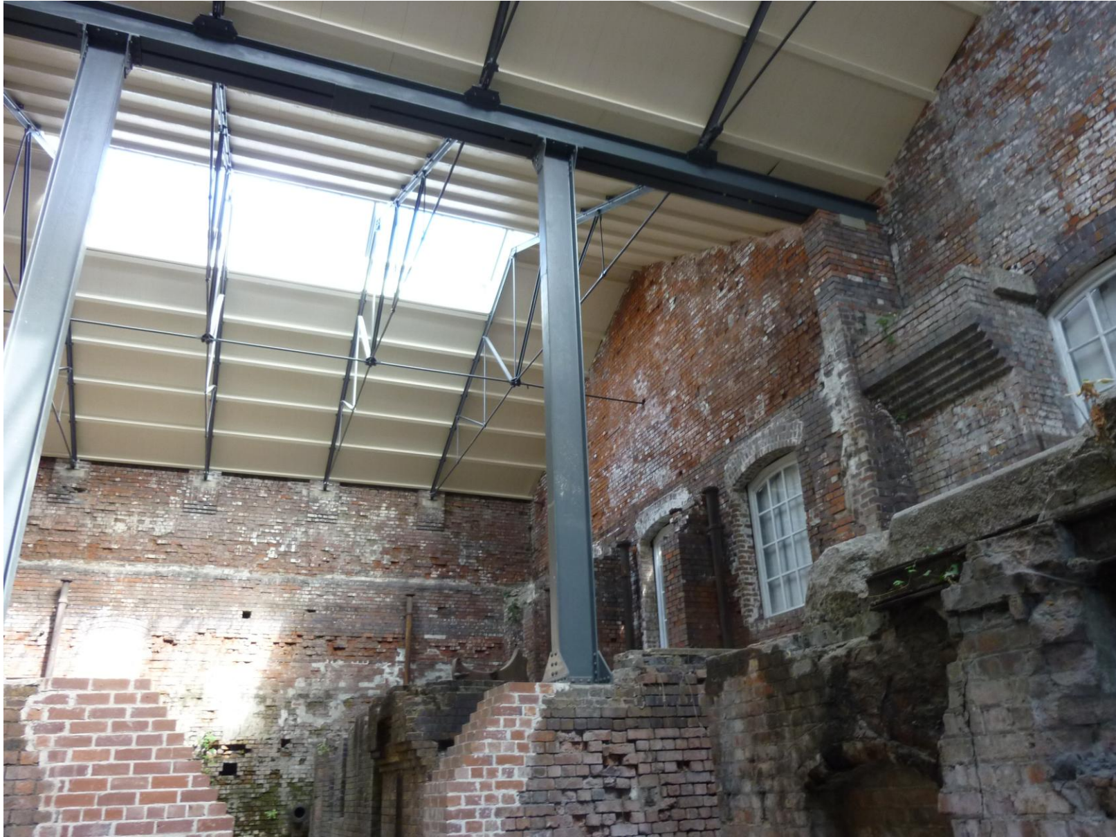
PH22 – east wall of South Range
