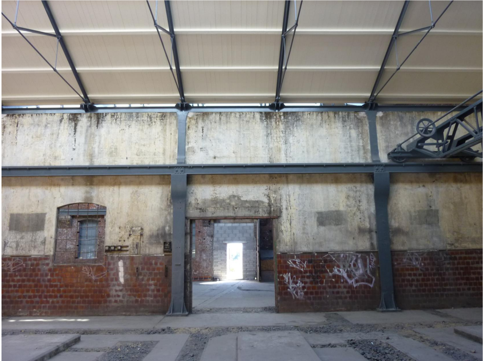
DH15 – internal wall of North Range from west
