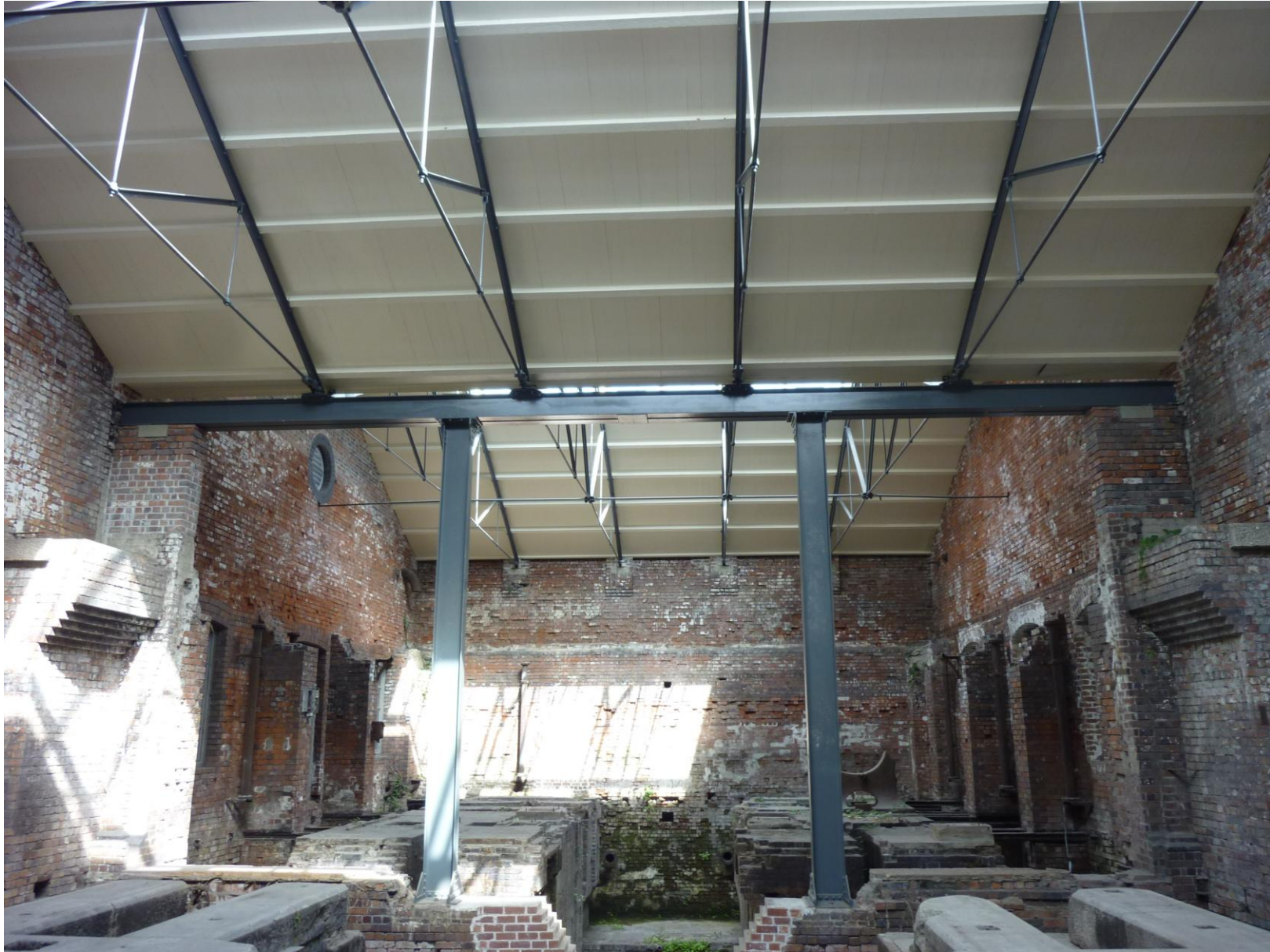
PF17 – north wall and machine bases in South Range
