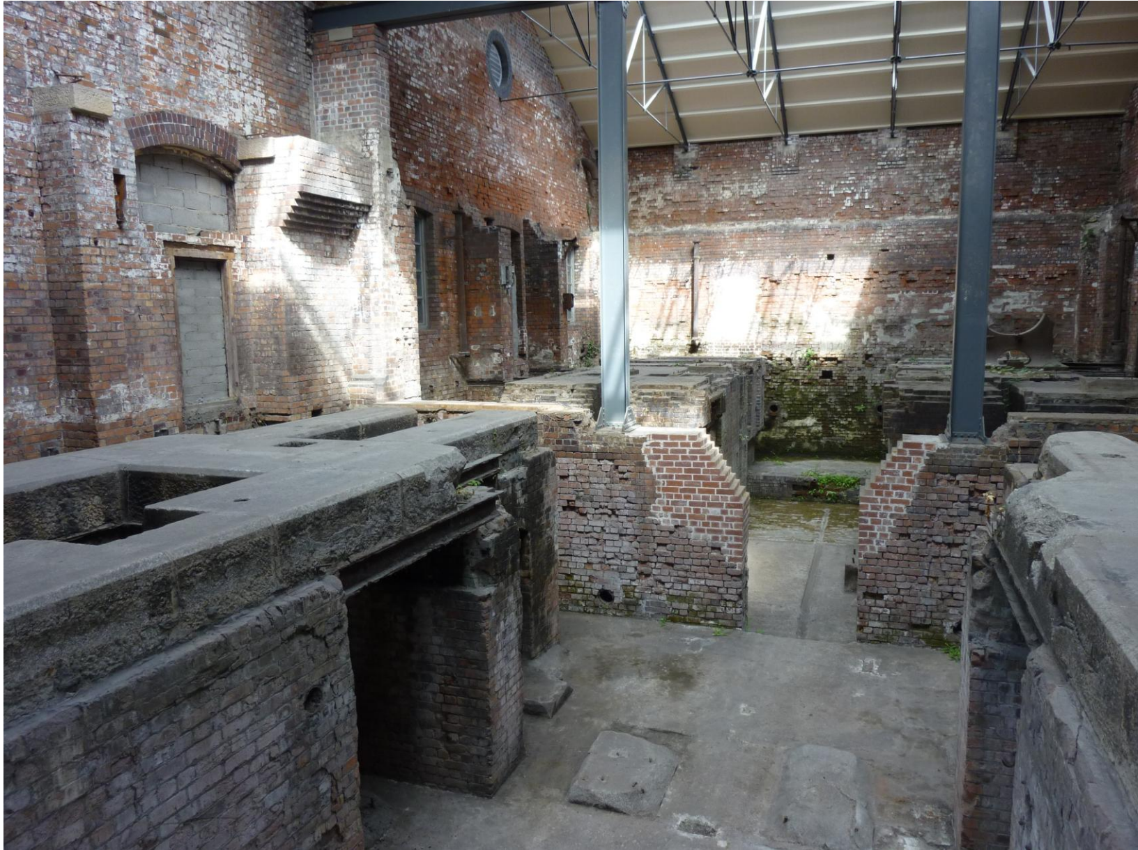
PH18 – machine bases in South Range
