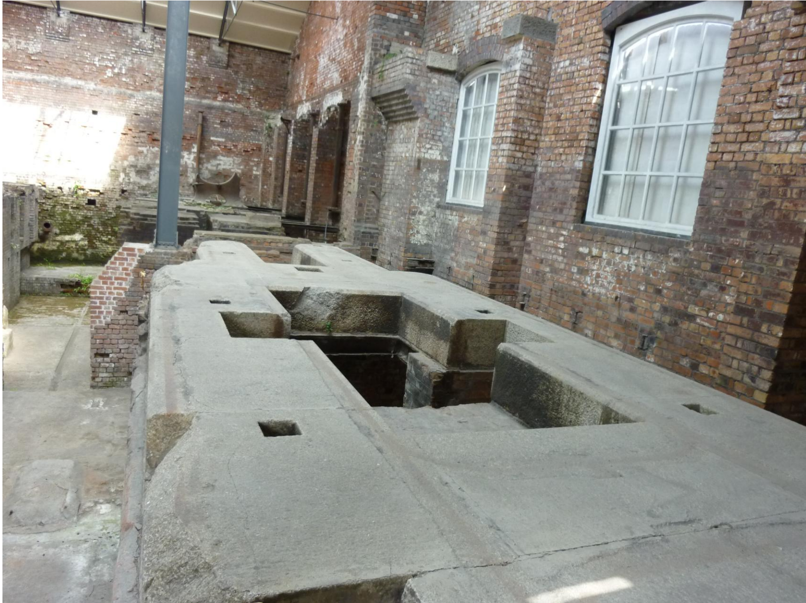
PH19 – machine bases in South Range
