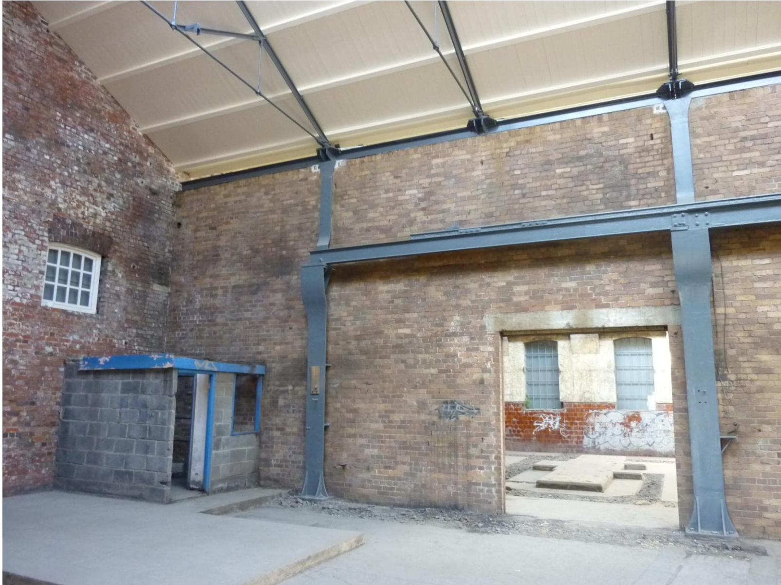
PH7 – the internal wall in the North Range from east
