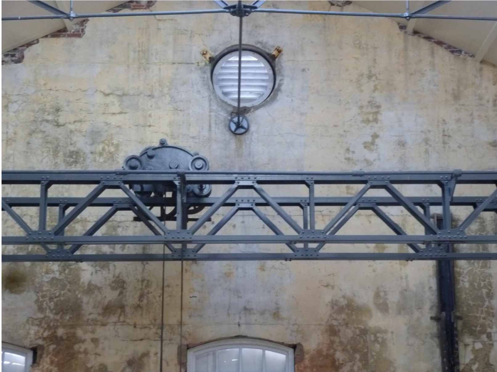
PH16 – crane support in North Range
