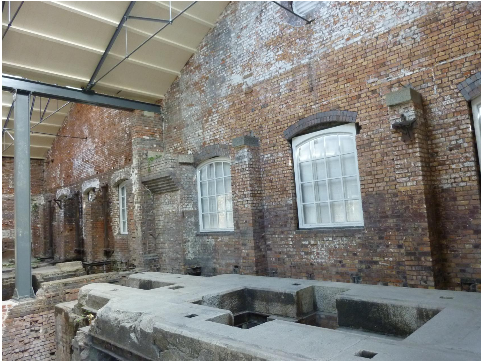
PH20 – east wall of South Range
