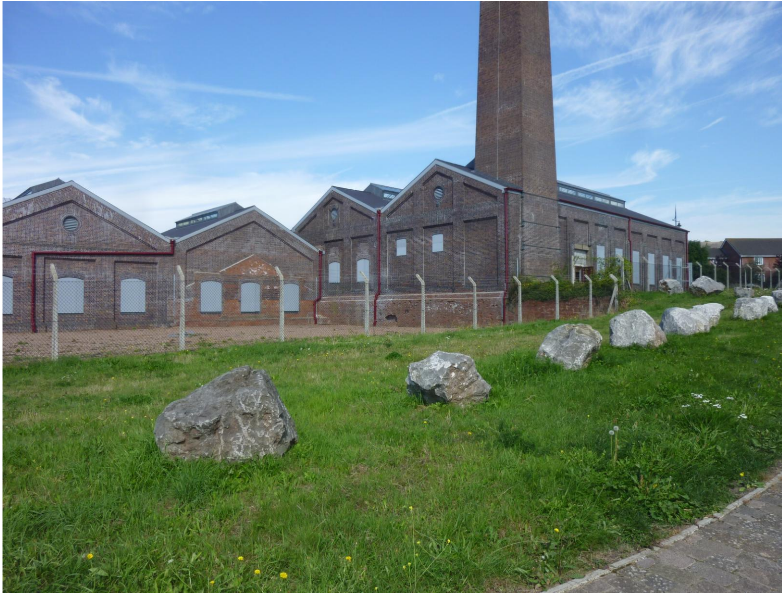
PH1 – the Pump House from the south east
