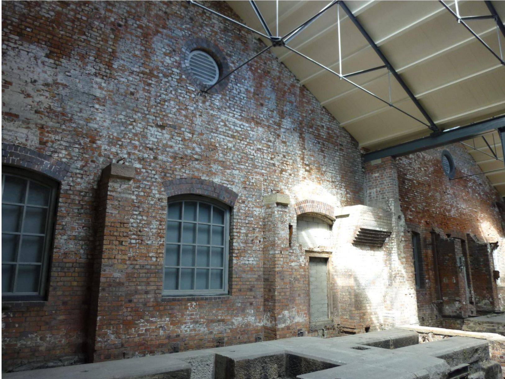
PH21 – west wall of South Range
