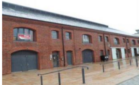
J Shed, Swansea
