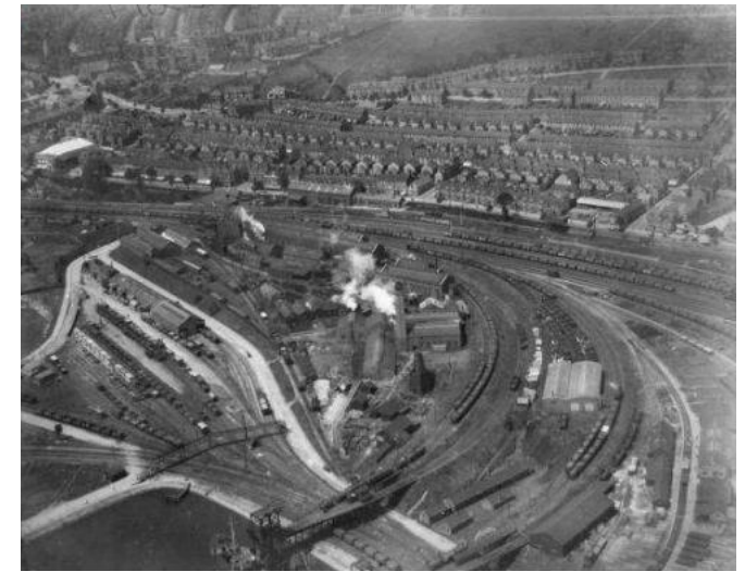
Aerial view with pumping station
