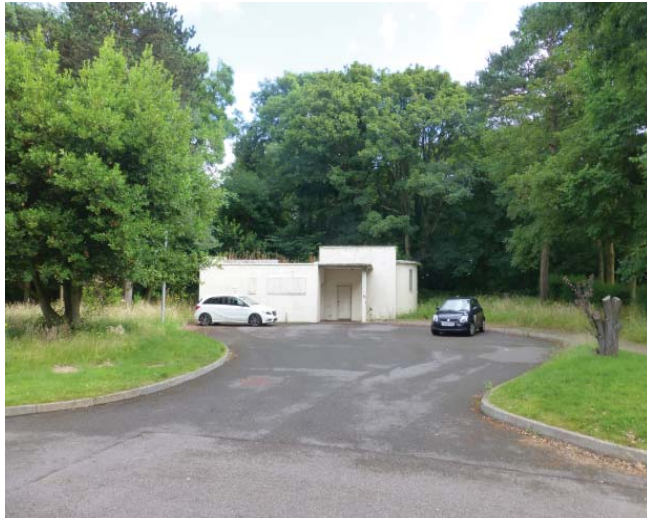
Photo 2 South elevation of existing building
