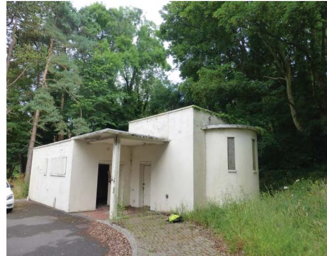
Photo 4 Existing canopied entrance
