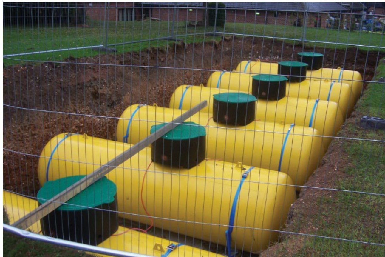
Photo 1: Underground tank installation
