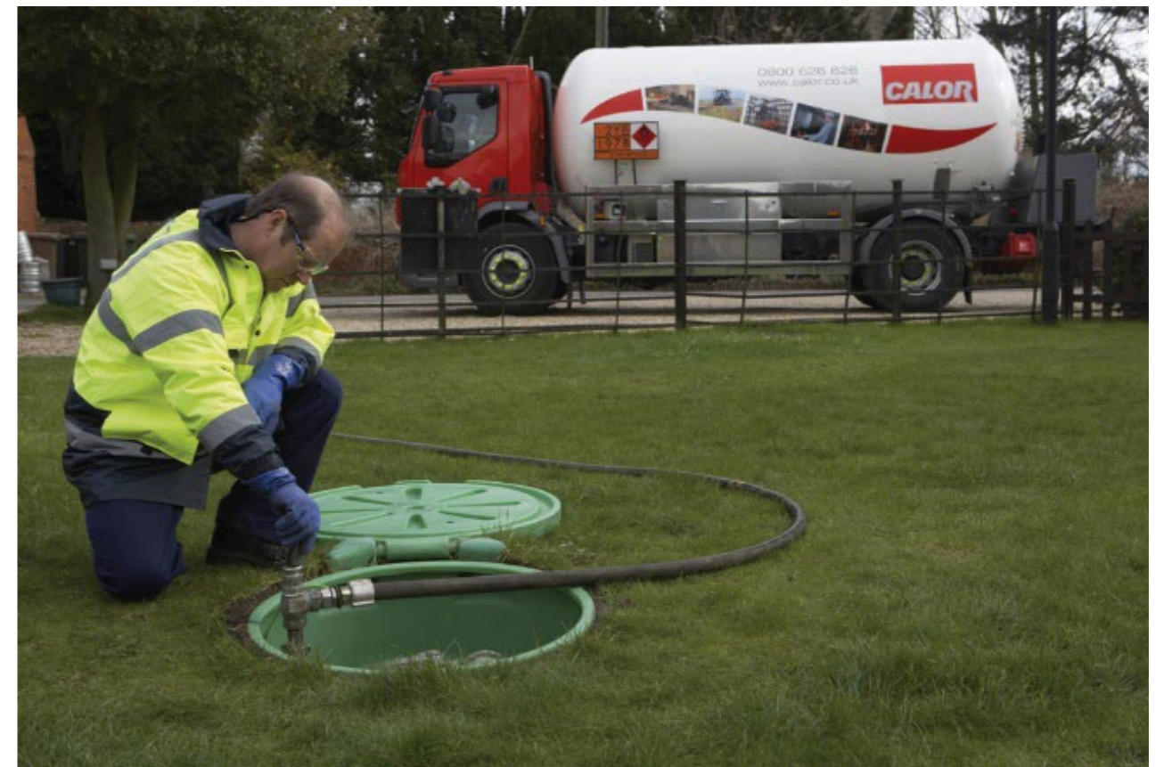
Photo 2 Inspection chamber cover at surface level.
